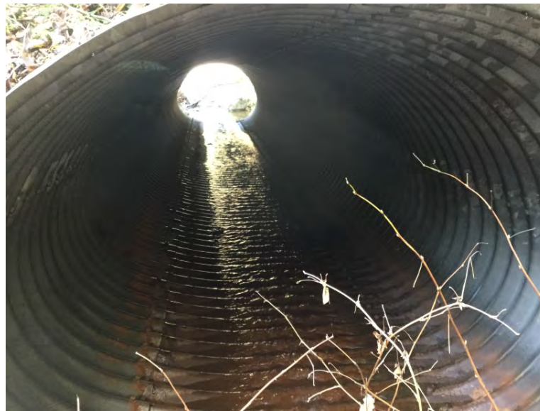
Looking through culvert from inlet
